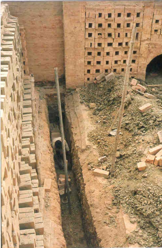
Trench for installing ground t/c
