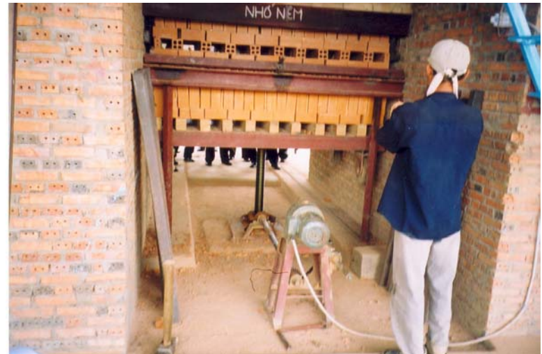
Hydraulic system for unloading
