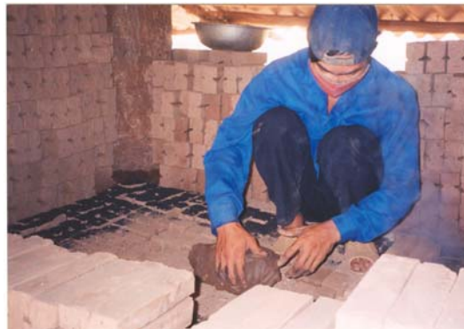
Loading of bricks and Coal feeding
