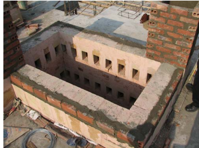
Factory made refractory flue ducts
