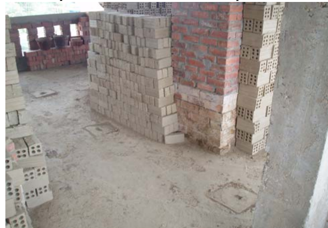
Holes for filling-up the insulation
